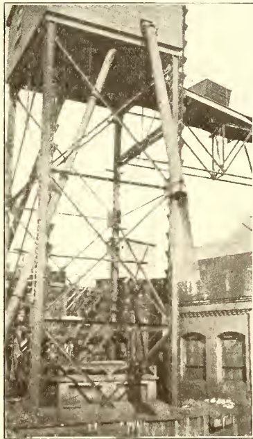
COAL AND ASHES HANDLING— COAL TOWER AND BUCKET CONVEYOR, SPRINGFIELD PLANT
